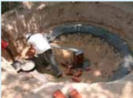
In the Indian province of Tamil Nadu around 900 dome furnaces are being built, in which farmers ferment their cow dung. The resulting biogas is piped into their houses as fuel for simple gas cookers.
