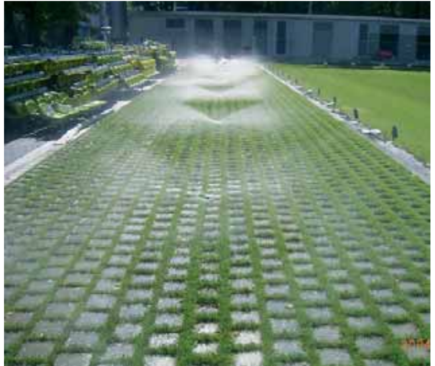
In order to limit sealed areas as much as possible, grassed gravel and concrete paving was employed, which lets water seep away.
