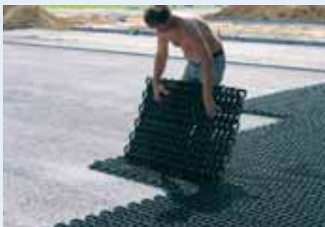
Many stadium car parks are paved with water-permeable materials. In Cologne, lattice mats made of recycling plastic were employed.
